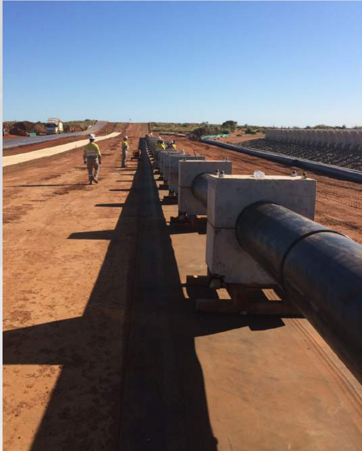
Kiewit Onshore to Offshore Pipe Transport Bogies
